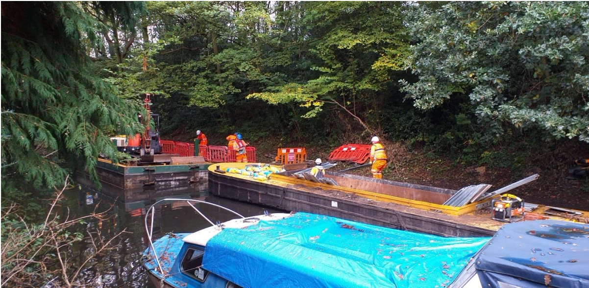
Taking out the old piling
