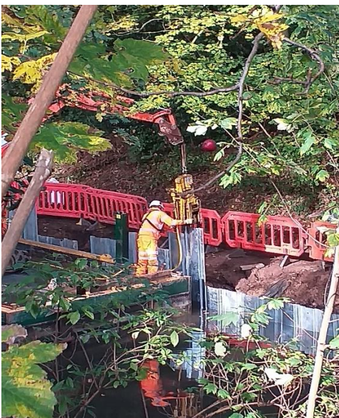
Piling removed, old piling can be seen on canal bank
