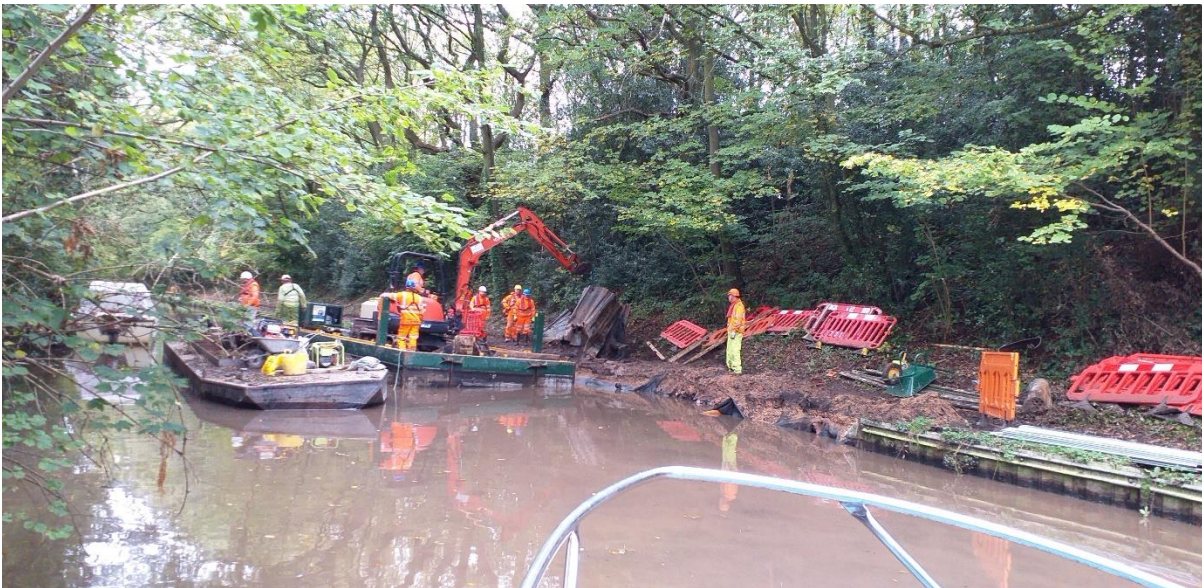
Piling removed, old piling can be seen on canal bank
