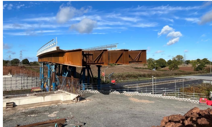
Bridges driven across M42 to avoid using tall cranes
