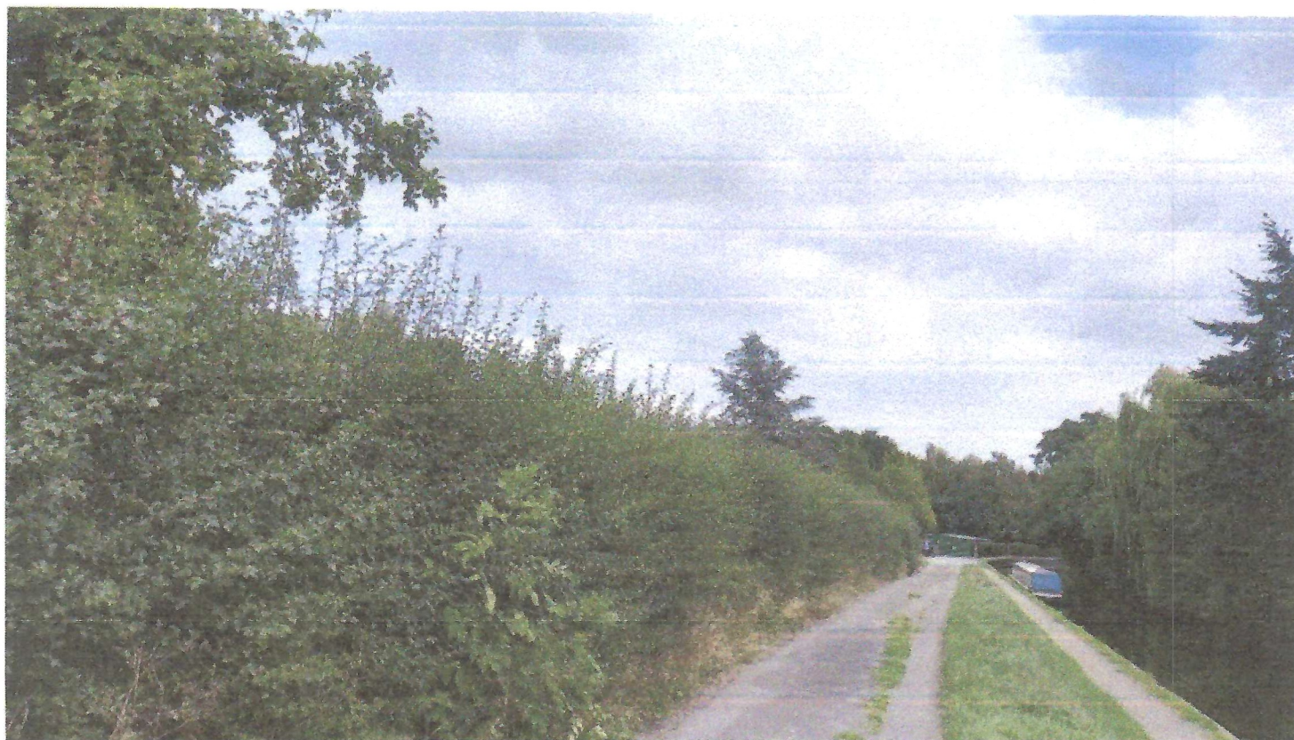
Current view along canal from the B4102 bridge
